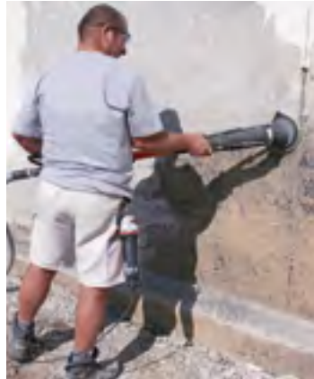
Grinding bitumen coating with PCD grinding disc
