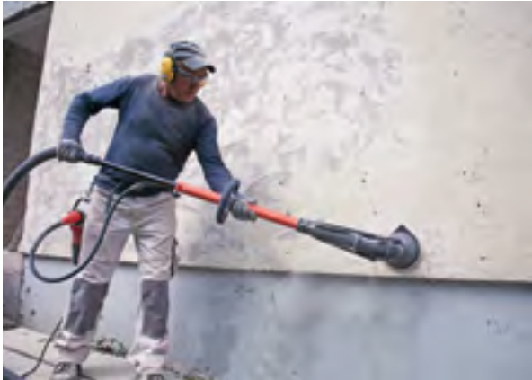
Removing old plaster and paints
