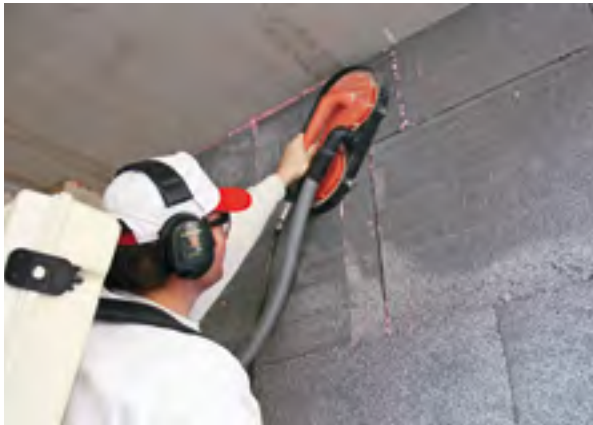
Grinding EIFS and ETICS boards
