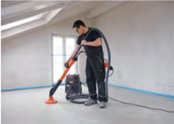
Grinding screeds
