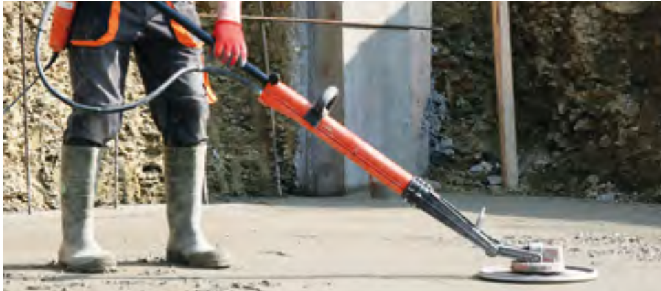
Levelling fresh concrete
