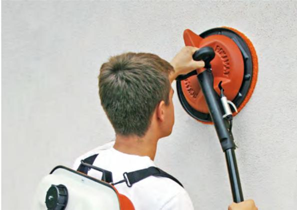
Sophisticated engine technology: Lower rotation speed possible → for a perfect surface structure
